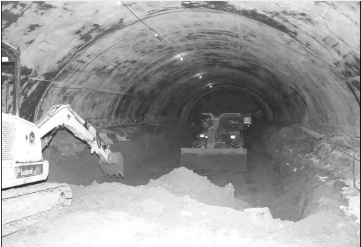
Fig. 3. "Belgian" tunneling method, Line H, 2000.
