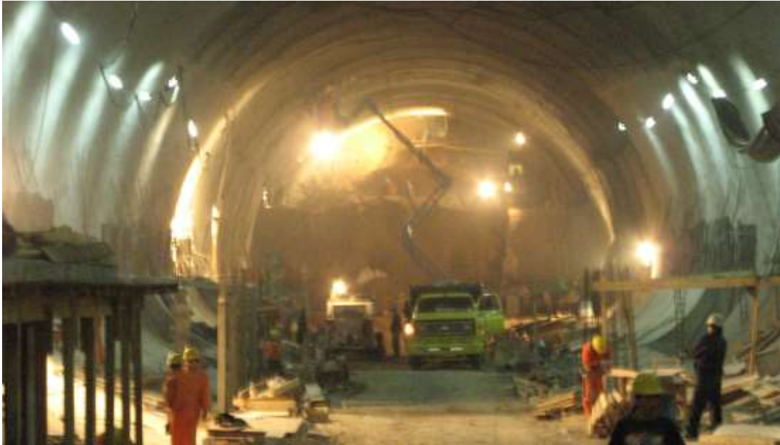
Fig. 9. Corrientes Station, Line H. Full face excavation.
