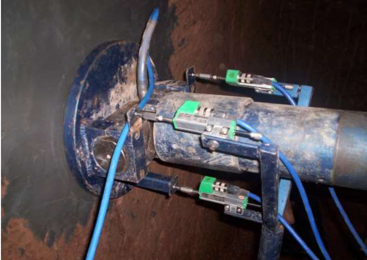
Fig. 5. Plate load test, Line B, 2006.
